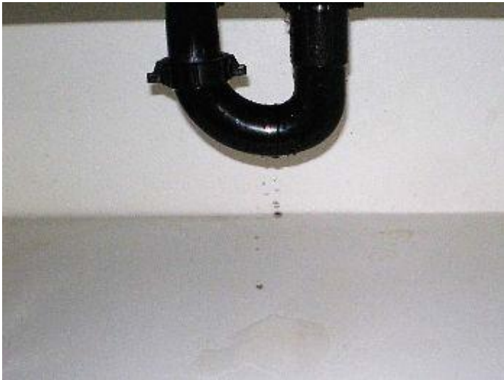
Water leaking from Bathroom #2 Left
