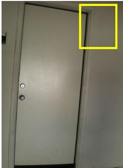
Absence of self closing device on Fire Door
