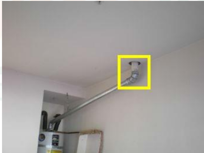
Water Heater Vent Pipe at Ceiling Penetration
