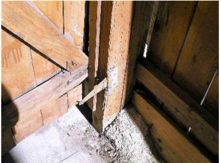
Gate - Lower Hinge - separated from door.
