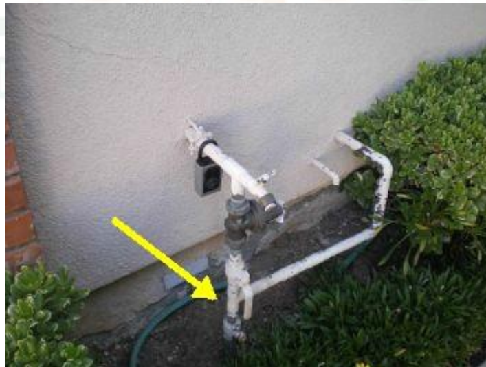
Main Water Shut Off at front Walkway
