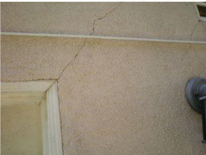
Representative sample of hairline cracks observed.
