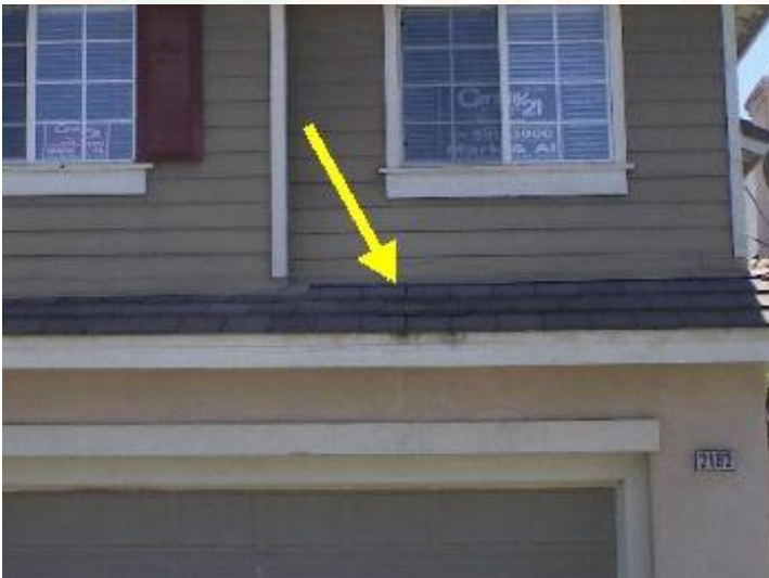
Location of observed damaged shingles
