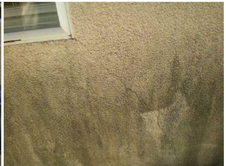
Representative sample of visible staining at exterior walls
