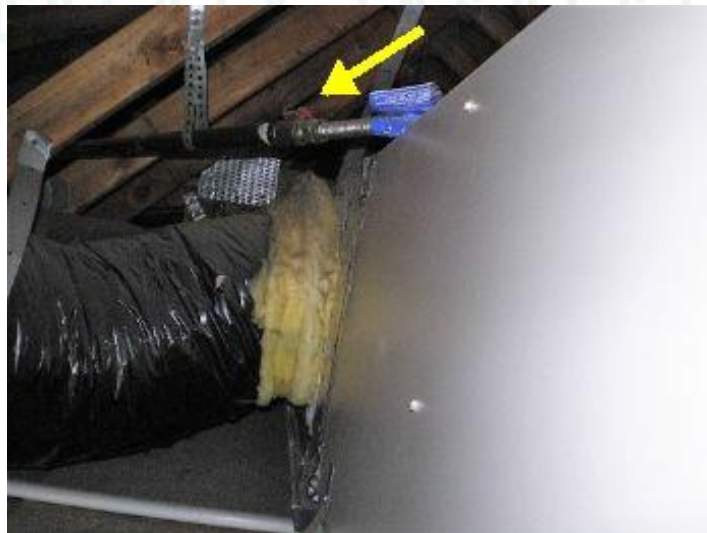
Emergency Gas Shut Off for Heating Unit
