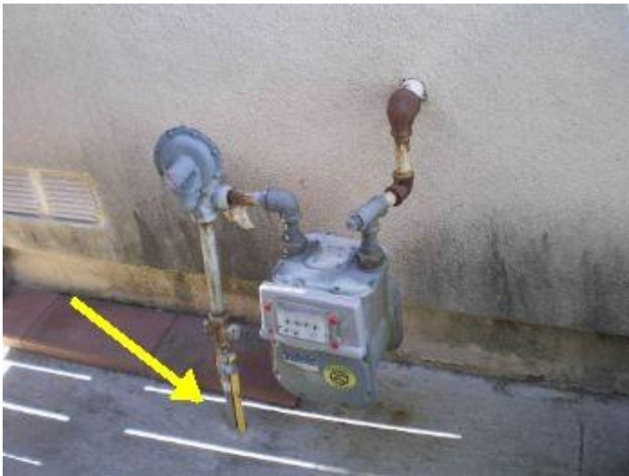
Gas Meter - Main Gas Shut Off Exterior North West of House
