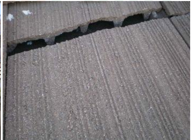
Cracked Roofing Shingle
