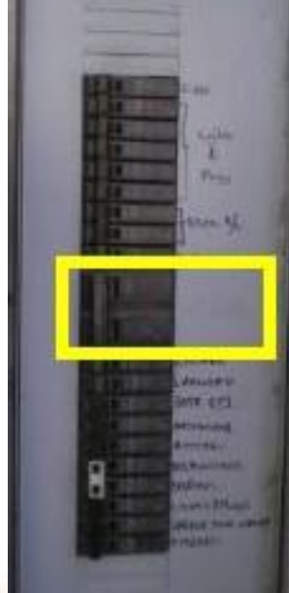
Fuse Box - Main Disconnect Breaker
