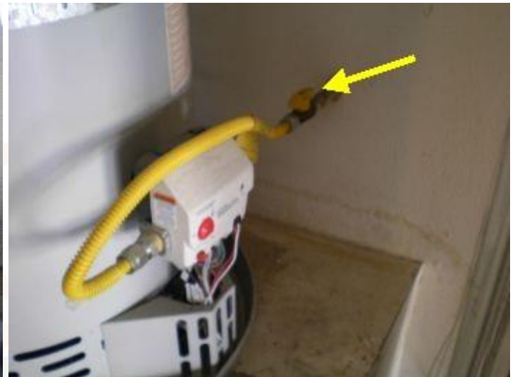
Water Heater - Gas Shut Off - Garage
